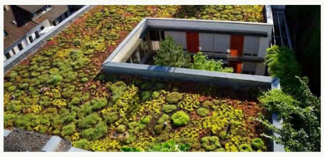
room2 Chiswick's roof stores 50,000L of water that is slowly drained to mitigate against local flooding.
